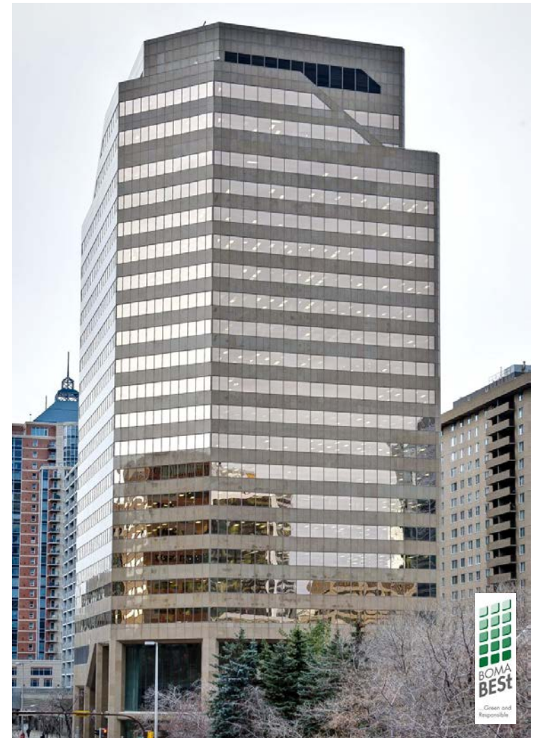
Trimac House – Calgary, AB
